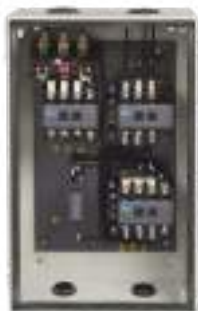
Interior View of MU FASD
